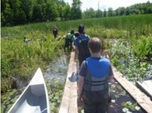
Volunteers and staff combine efforts to transport materials to remote build sites. Photo by Jérôme McDuff.
